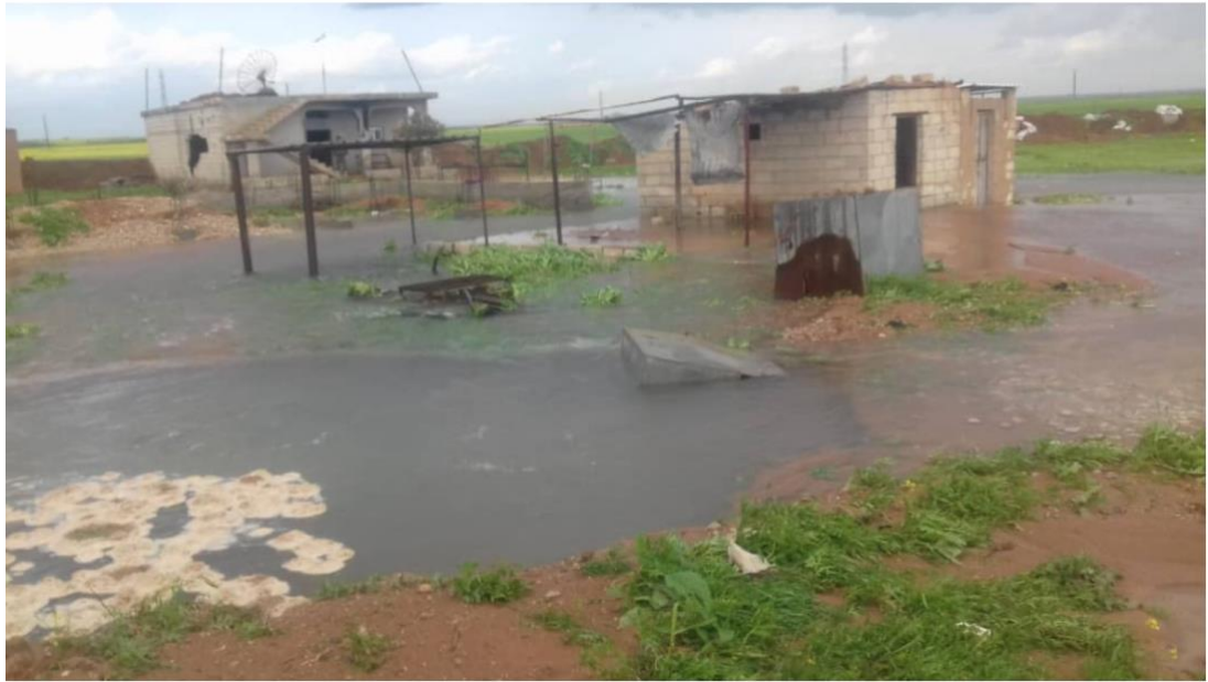
Wasted water after Turkey shells water pipes, 2 April 2020
